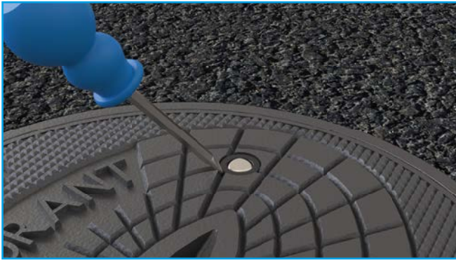
Remove the dirt gasket.
